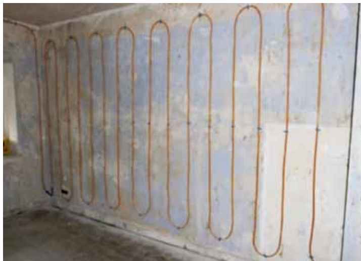
Figure 22: Wall heating system (Source: Heritage Department Hamburg)
