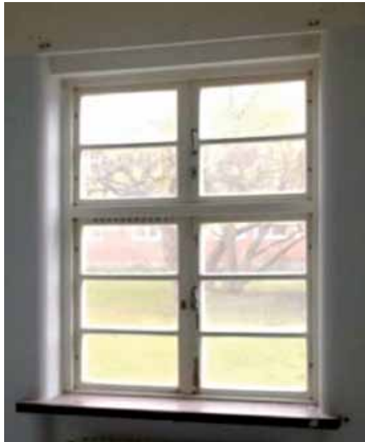
Figure 2: Existing window from the building studied
